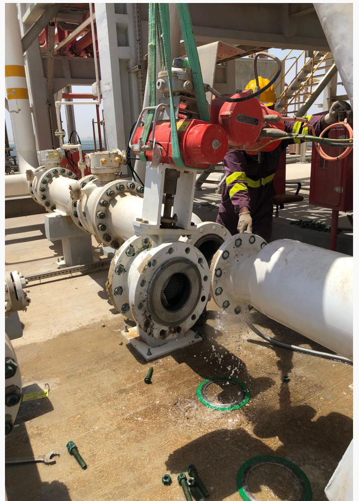
Pipeline Maintenance Activities
