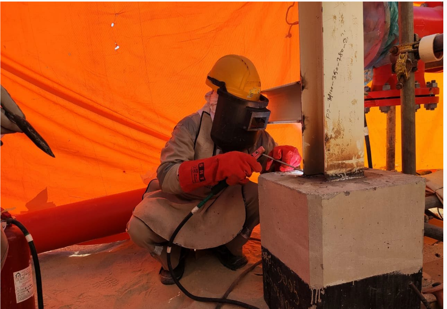
Welding Activities On Structures
