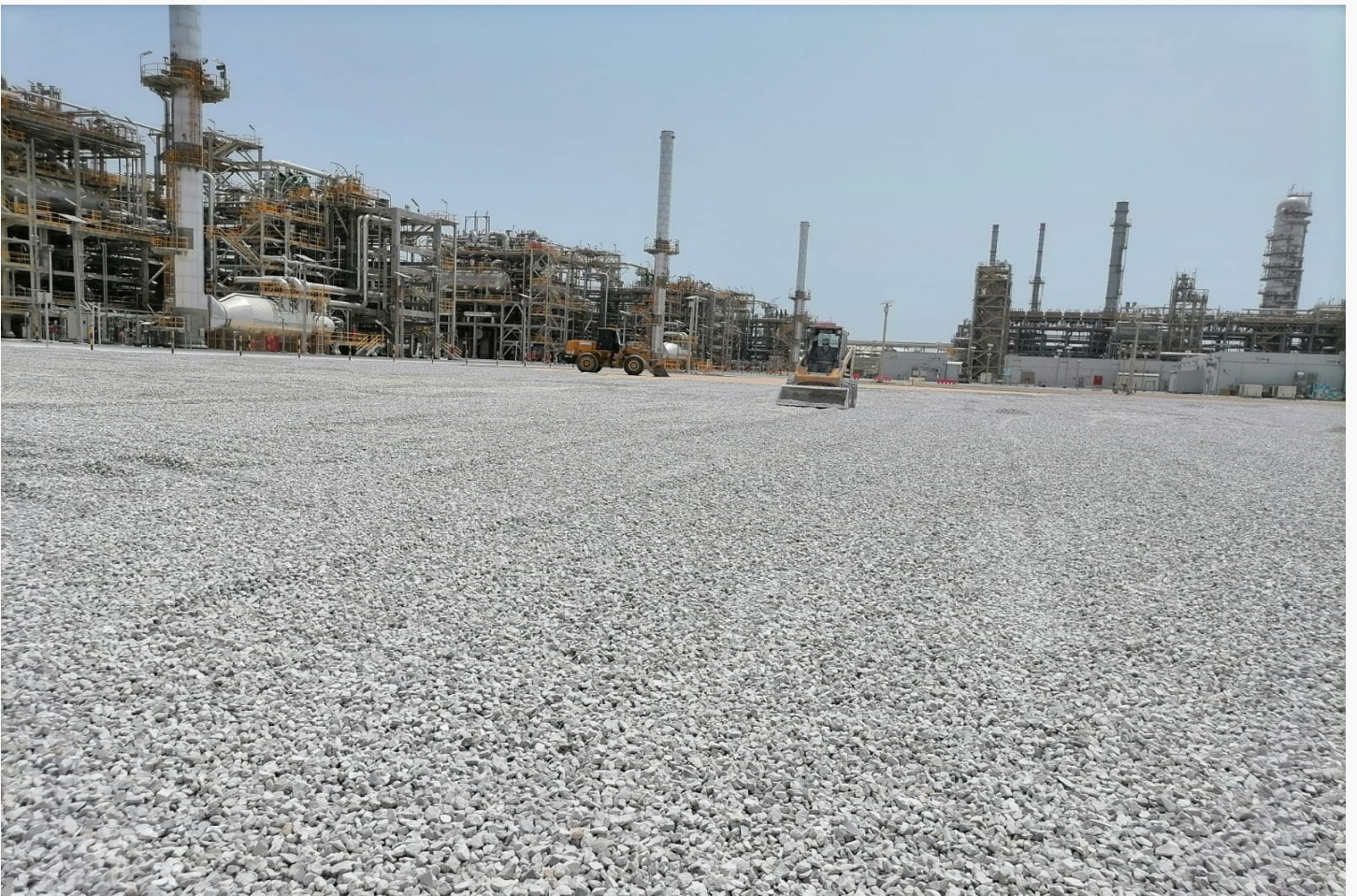
Gravel Laying Work In Duqm Refinery
