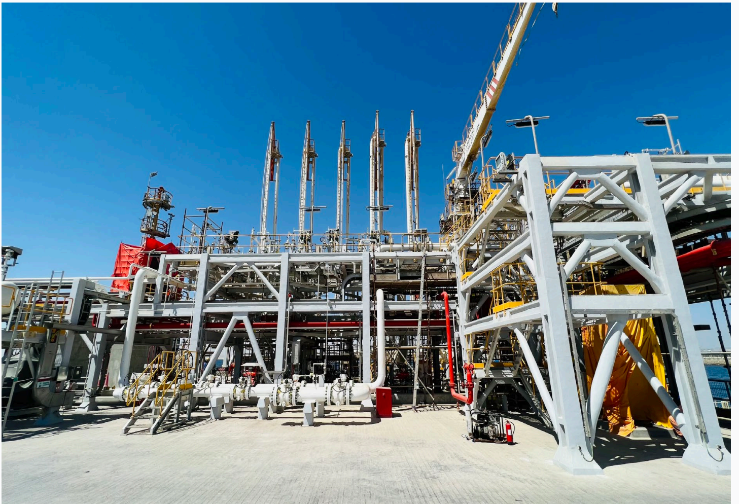
Fireproofing Application On MLA's
