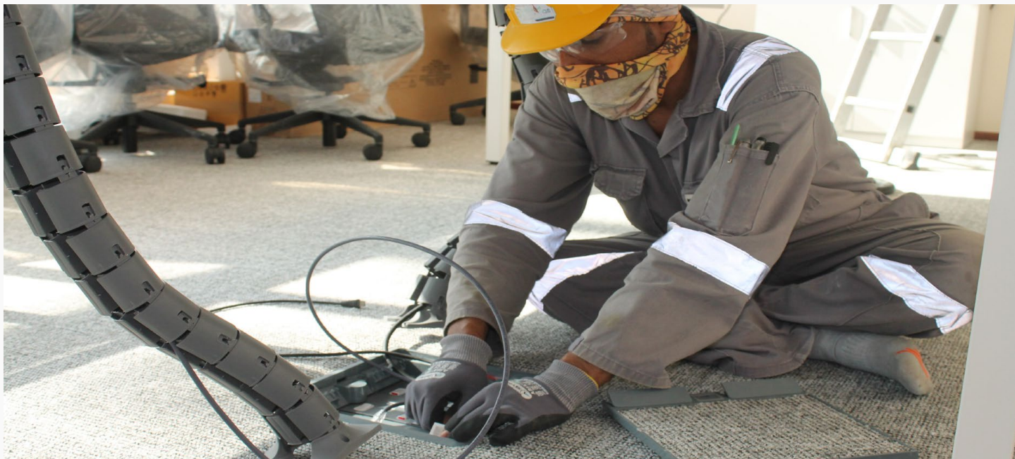
Floor Box Fixing
