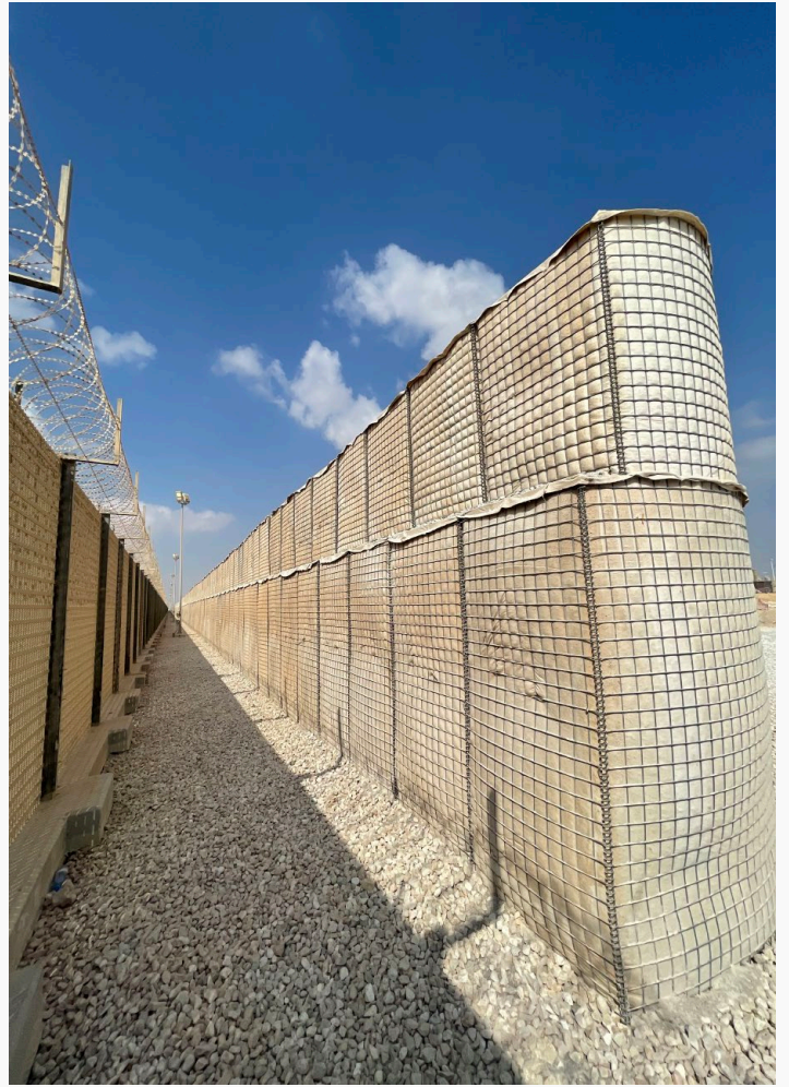
Installation Of Hesco-Rapid Deployment Barriers
