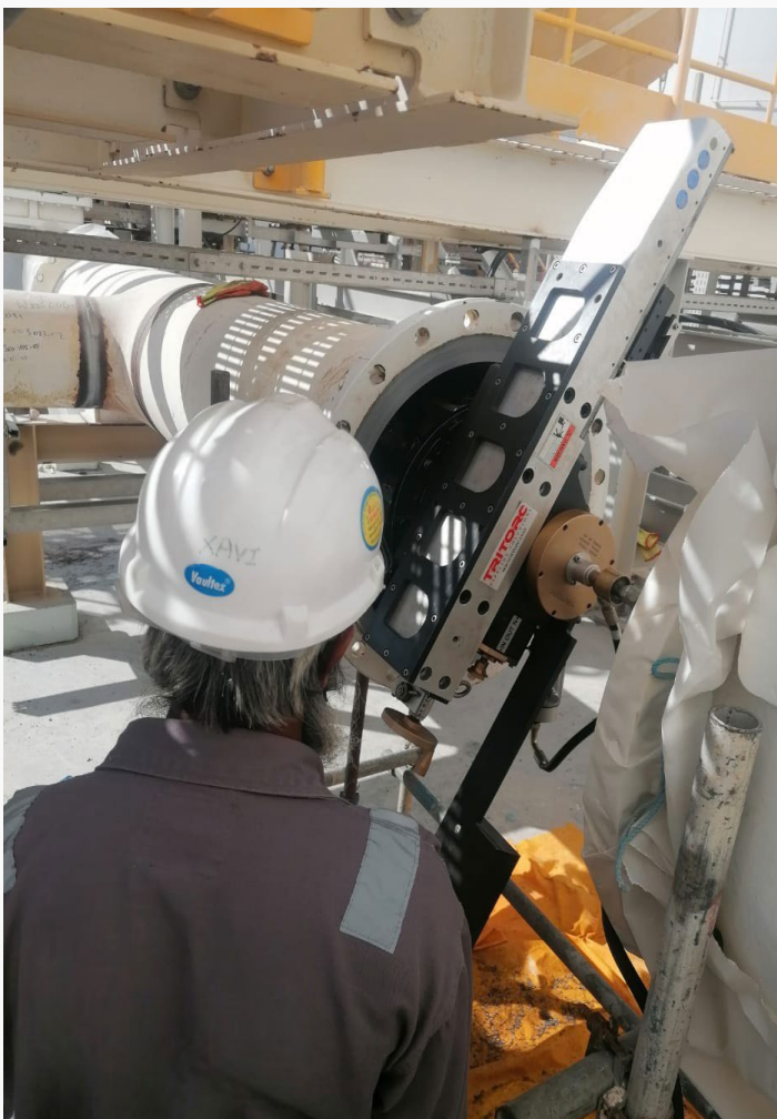
Flange Facing For GRE Pipes
