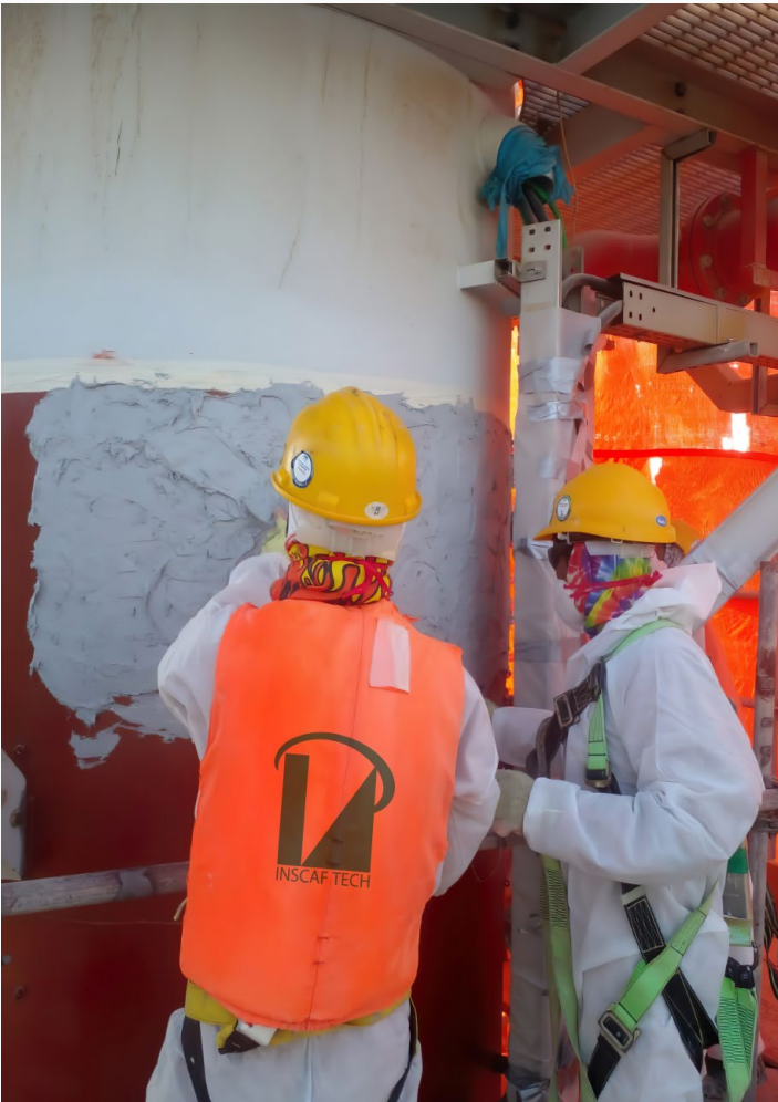
Fireproofing Job(Intumescent Coating)
