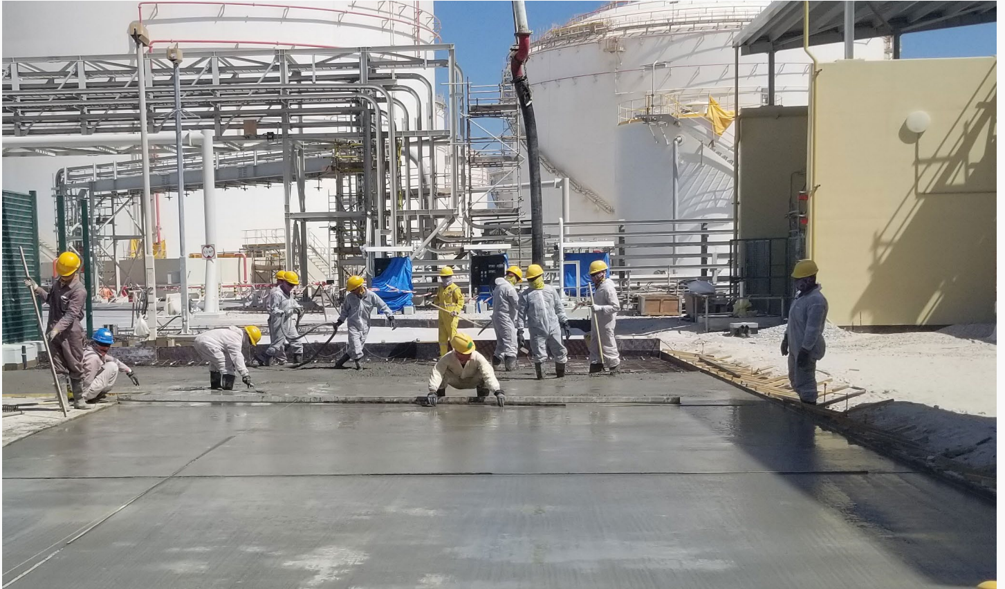
Floor Concrete Work
