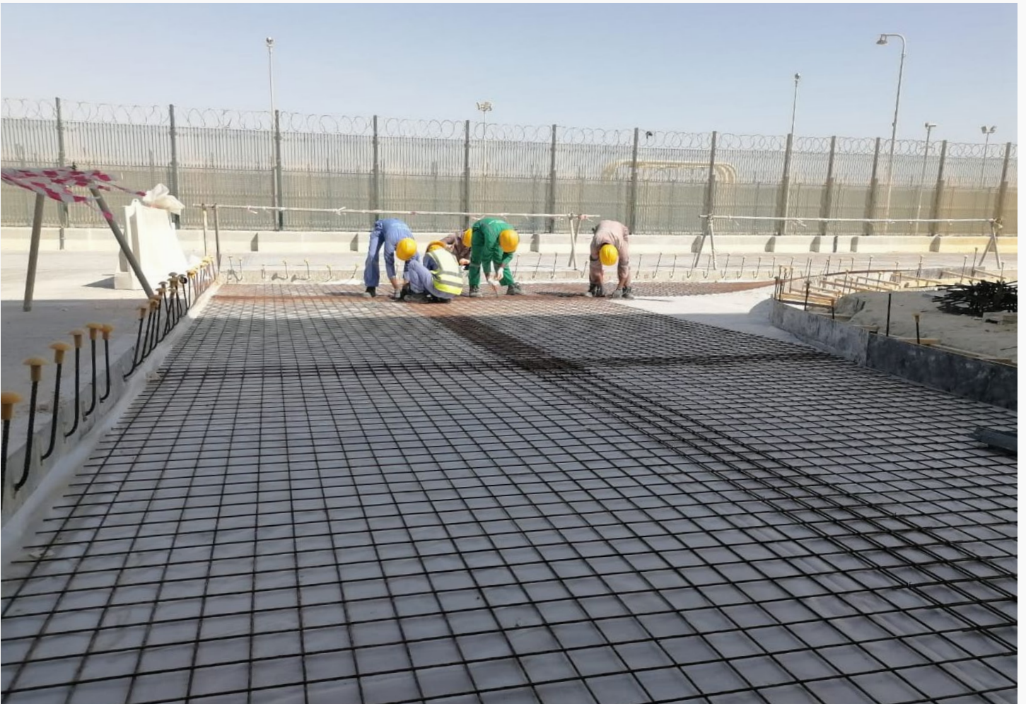
Shuttering and Steel Fixing
