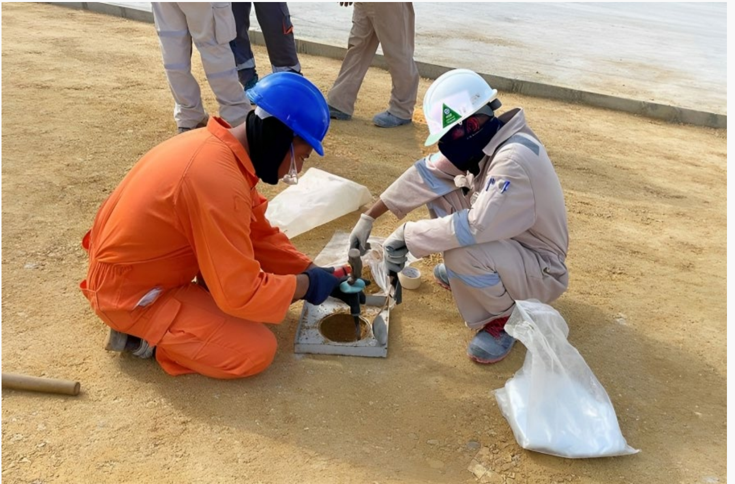
Soil Inspection Work
