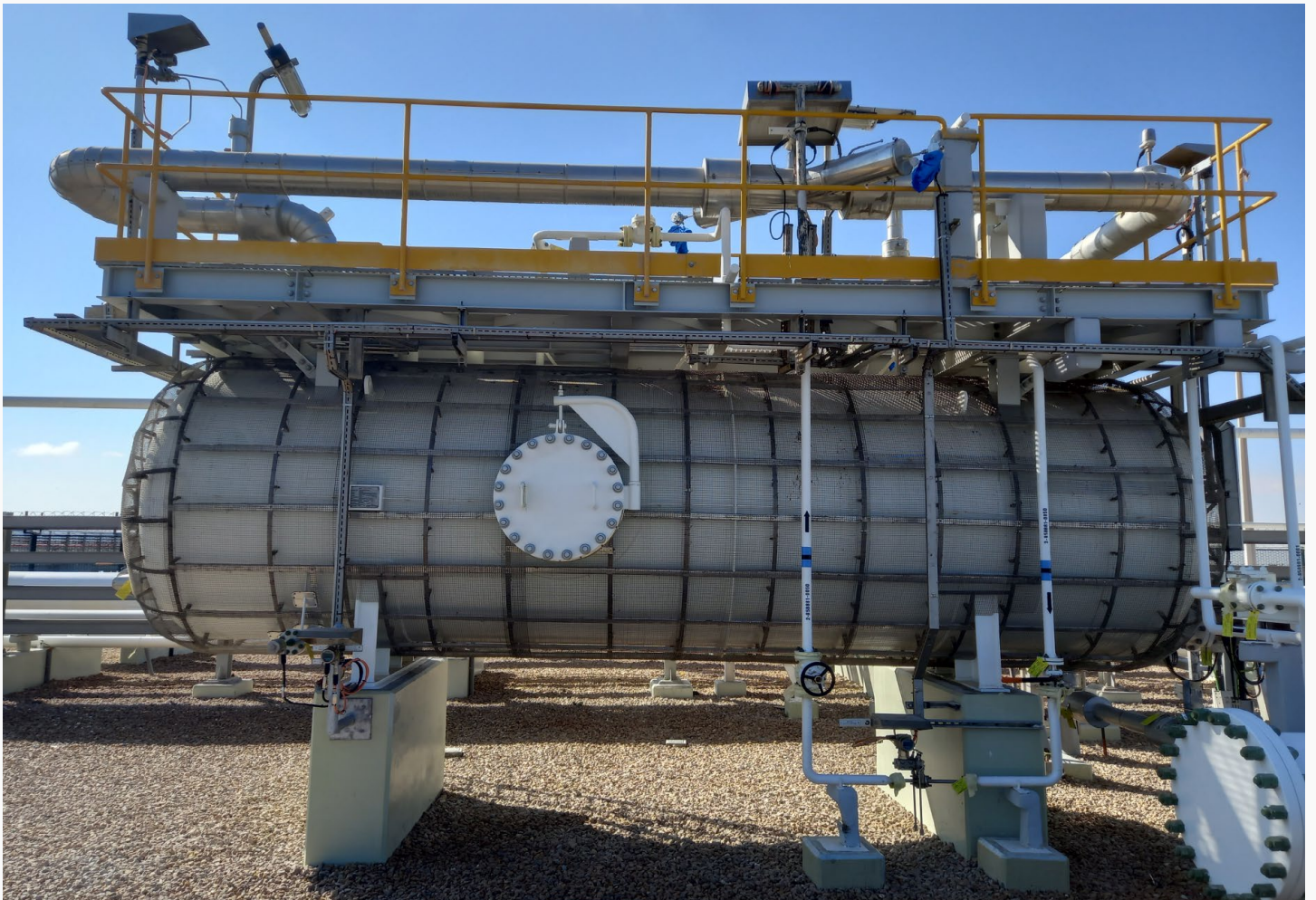
PP Insulation On Flare Knock Out Drum
