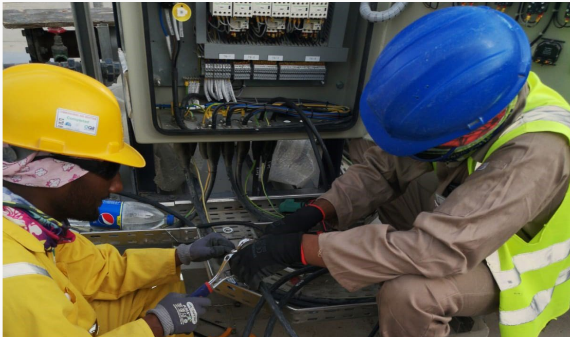
Cable Glazing & Termination Works
