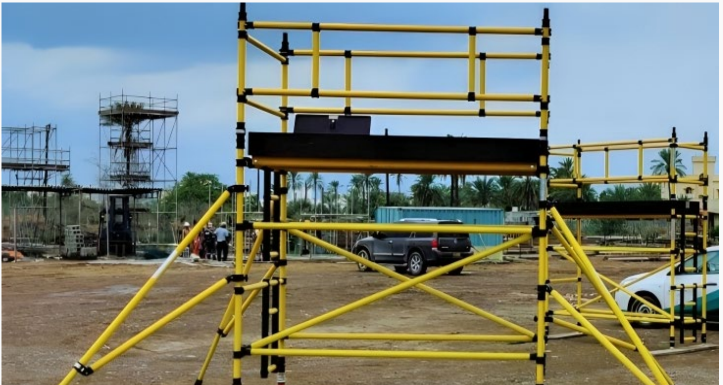
Fibre Glass Scaffold
