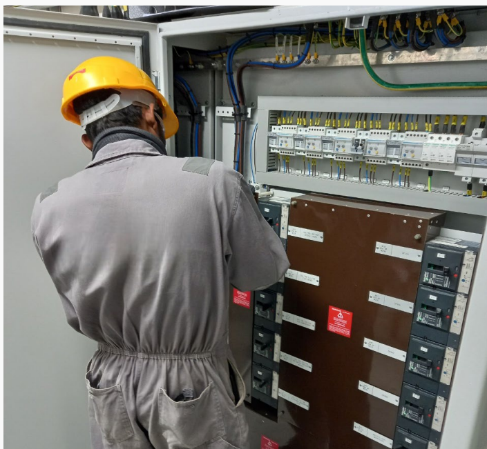
Lighting & Small Power Panel Cables Termination
