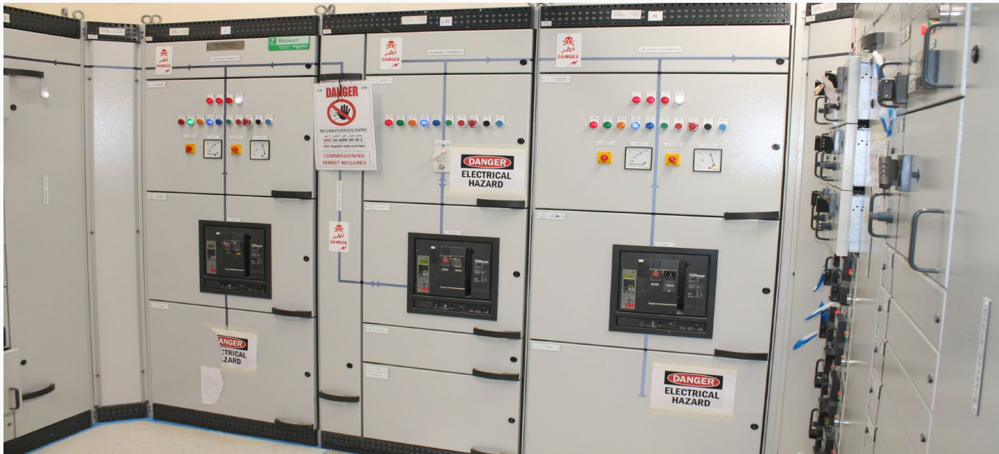
MCC Panel Installation & Cables Termination Work
