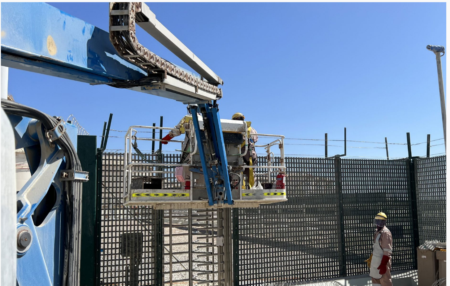
Security Razor Coil Installation For ROP 1min, 10min and IAPS Fence
