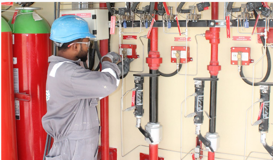
Fire Suppression System Accessories Installation
