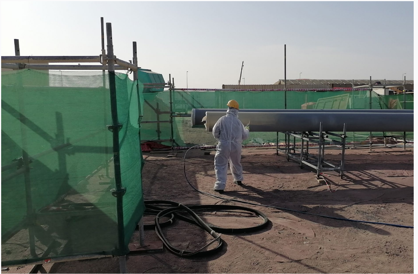
Spray Painting For Pipelines
