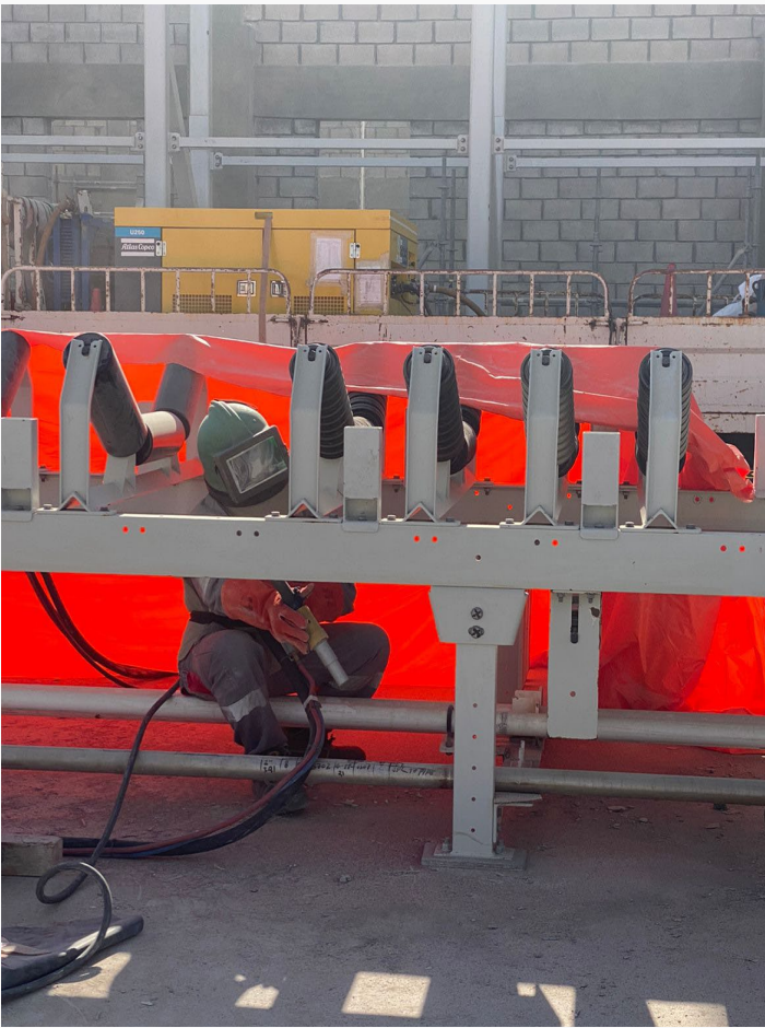
Installation Of Conveyor Structure
