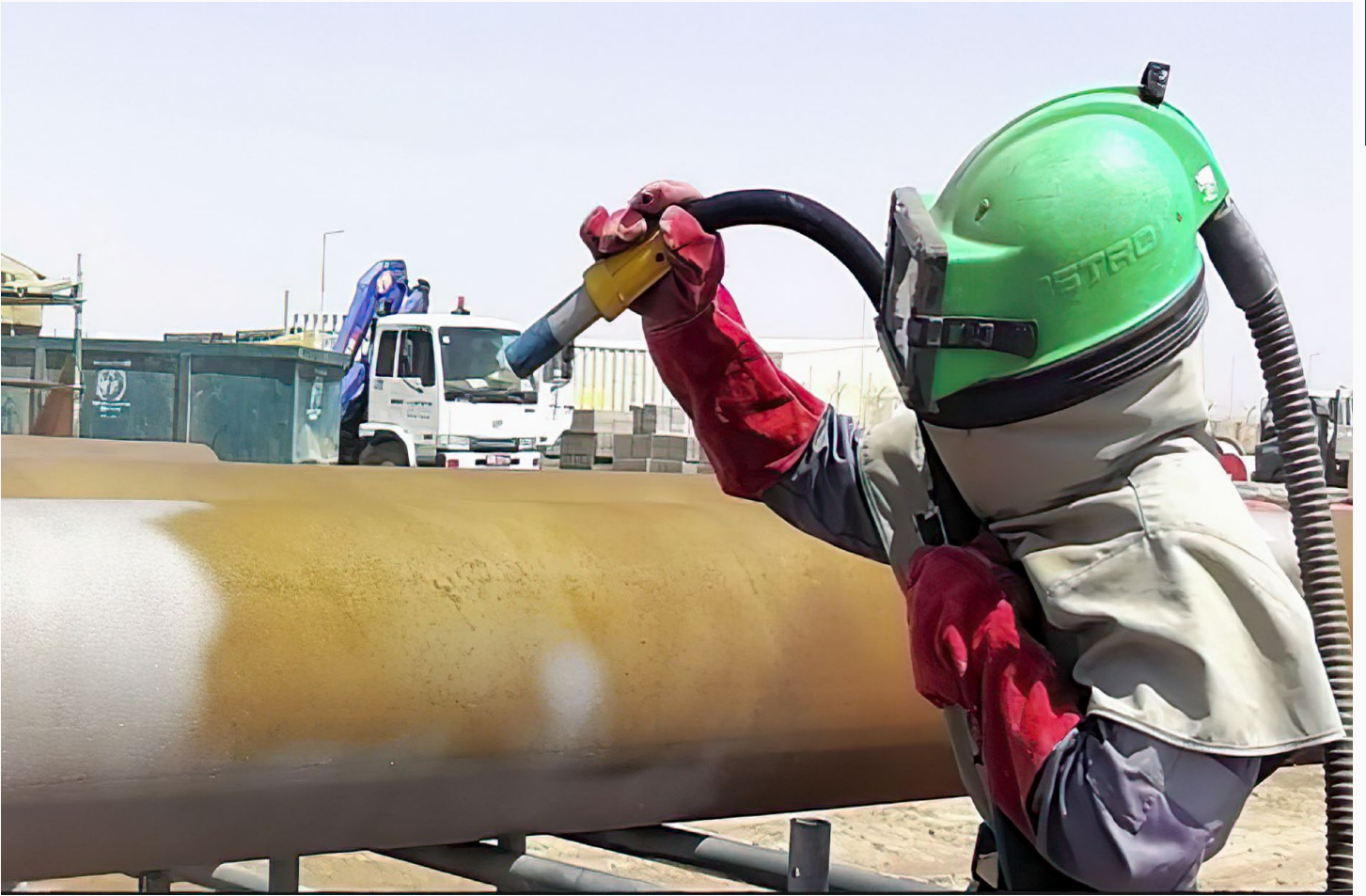
Pipeline Sandblasting Work
