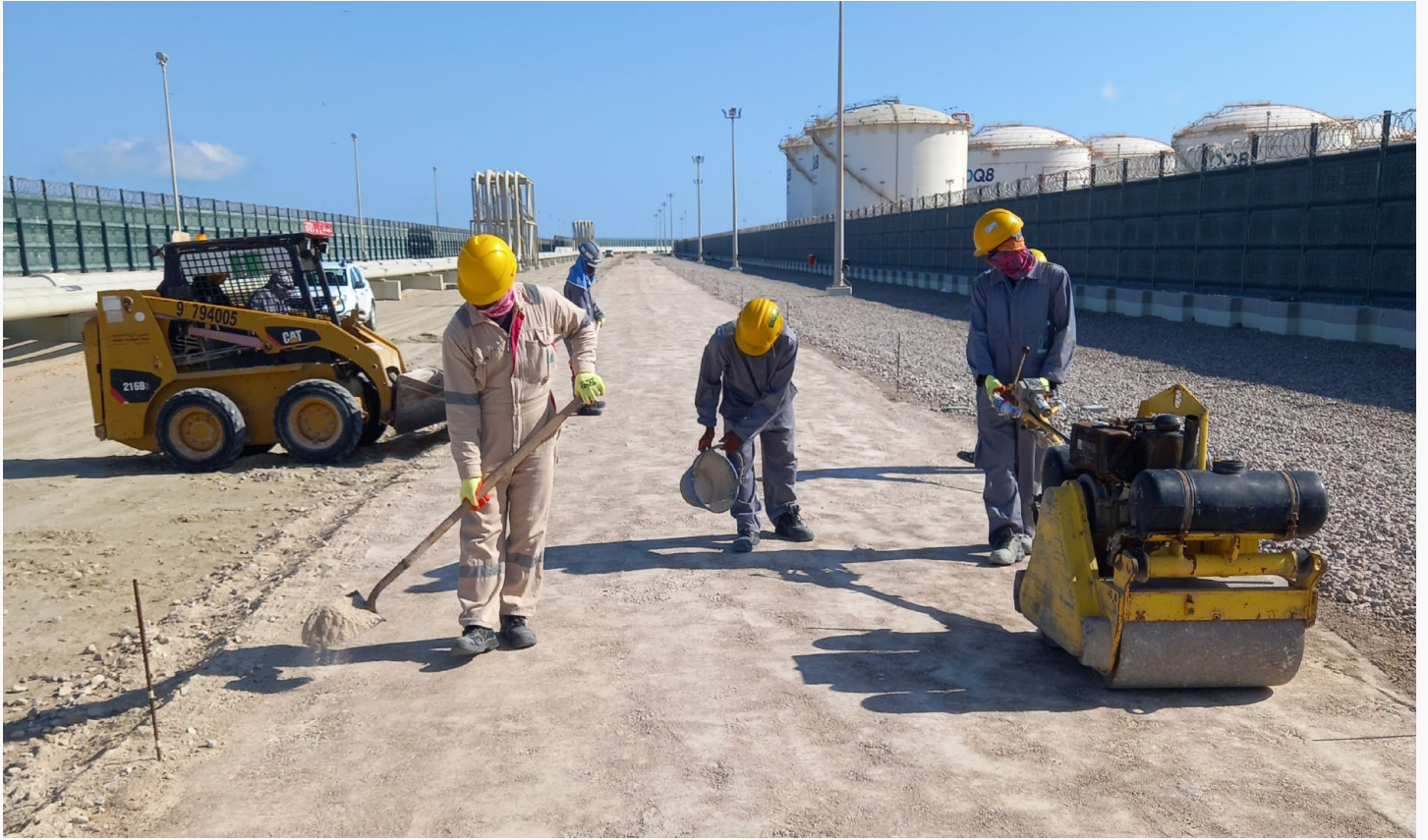
Road Work for Oil and Gas, Power Plant, Petrochemical Plant
