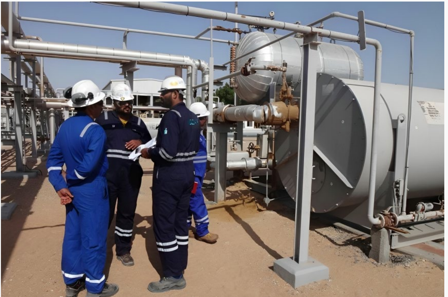
Inspection For Hot Oil Heaters
