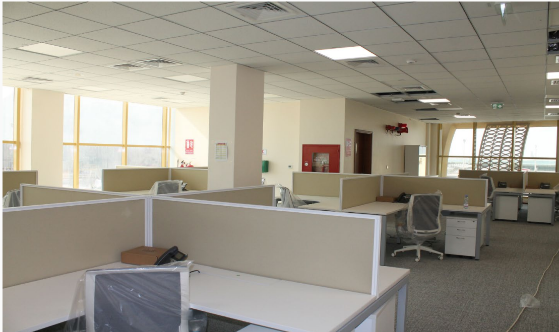
False Ceiling, Furniture, Floor Carpet Installation & Glass Window Installation
